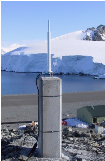
Figure 18 Concrete pillar on rock. (Rothera/ROTB)
