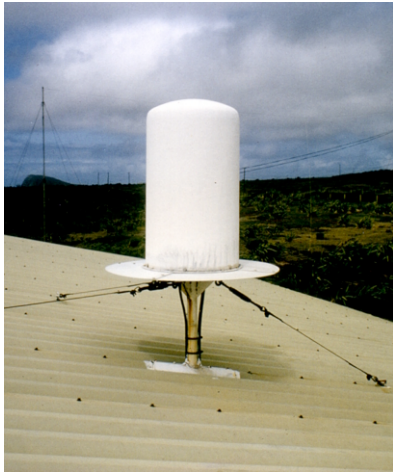
Figure 8: Antenna interface mounted directly on a roof ; no tower (St Helena/HELA)
