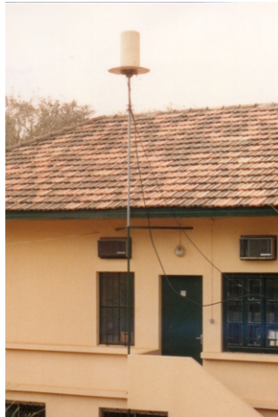
Figure 9: High steel pole, propped by very long guy-wires (Dakar/DAKA)
