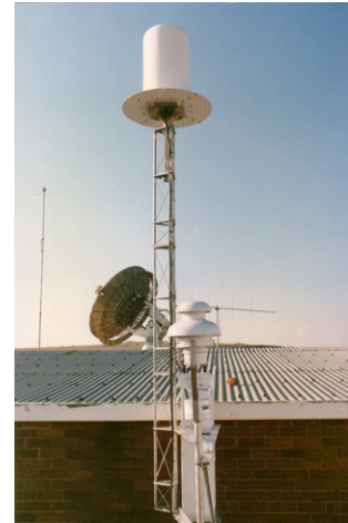
Figure 10: Side mount of a 3 m tower against a load-bearing pillar. No guy-wires... (Hartebeesthoek/HBKA)
