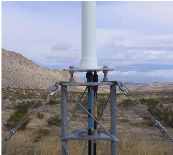
Figure 11 Base of the Starec antenna on a triangular plate mounted on top of a guyed lattice tower
