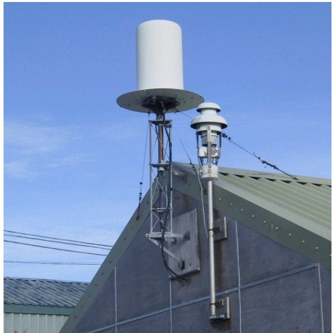
Figure 4: DORIS Alcatel antenna (left) on a one-metre tower and side wall mount. DORIS meteorological station on the right.
